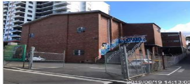
View of subject site from Hunter Lane
